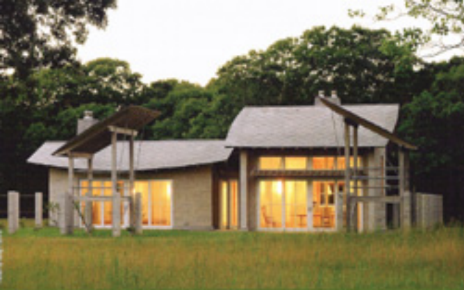
The greenhouse in Chittuck, designed by Kirk Mendow & based and coded by passive solar engineering. The wood-burning room is only supplemental heat.
